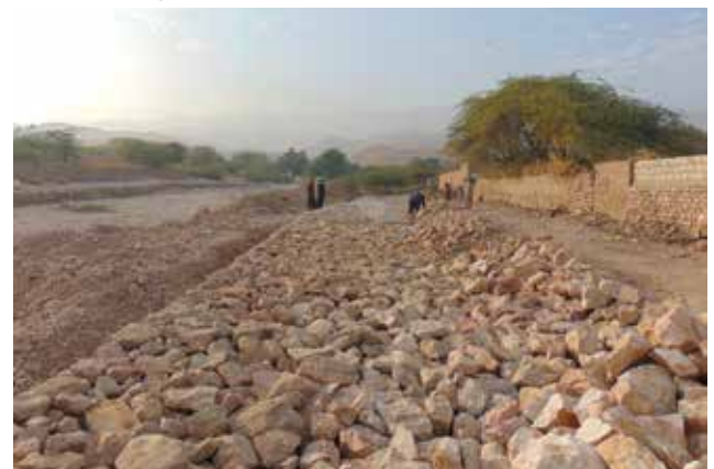
Figure.15: Incomplete flood protection structures were complemented by the project to prevent potential conflicts.
